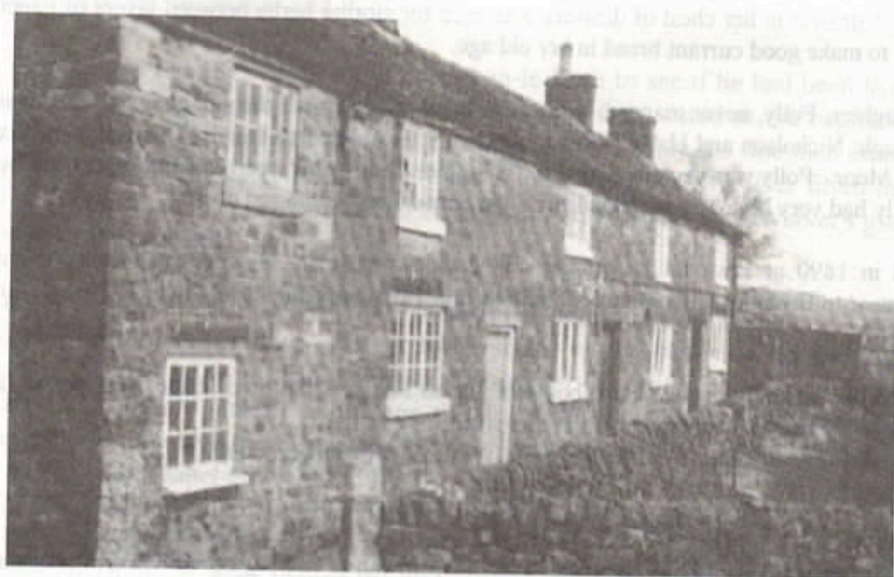
Lowe Hill Cottages, Leek, Staffordshire
