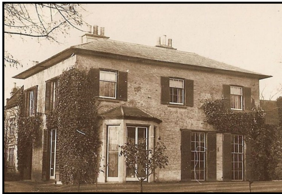
Risley Lodge. It later burnt down when in the process of being demolished
